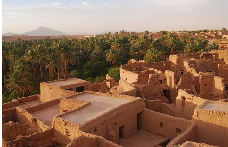
Fig. 2.2. The old architecture with raw earth in Adrar region.
