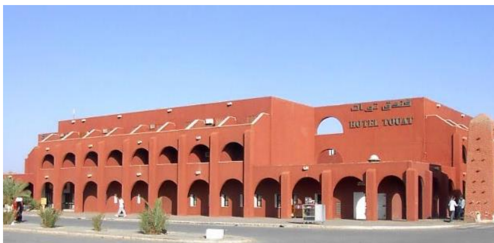
Fig. 2.1. New reinforced concrete architecture in Adrar region.
