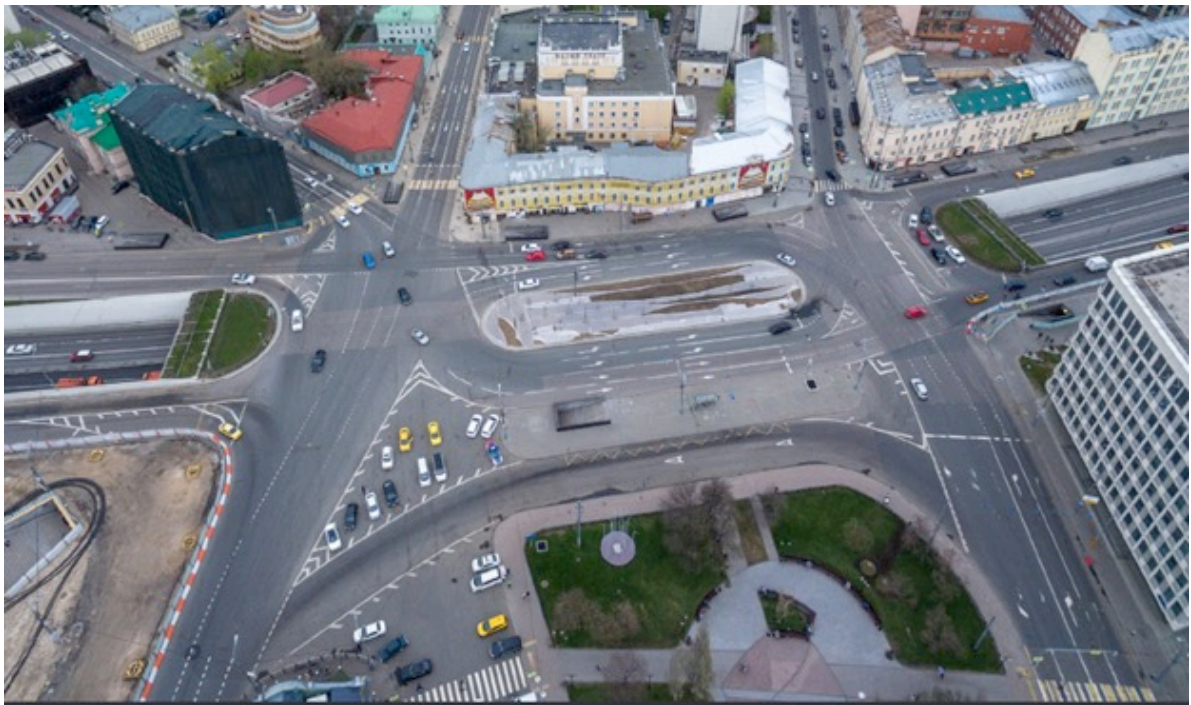
Fig. 3.3. Actual traffic organization of the road junction on Serpukhovskaya Square
